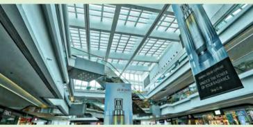
The solar film layer applied to Festival Walk's skylight helps to reduce energy demand for cooling the mall.
